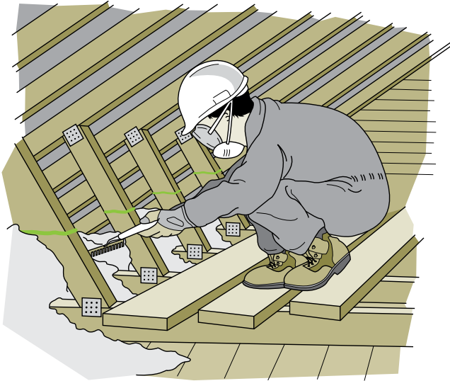
Figure 5-14 Installing loose-fill insulation
